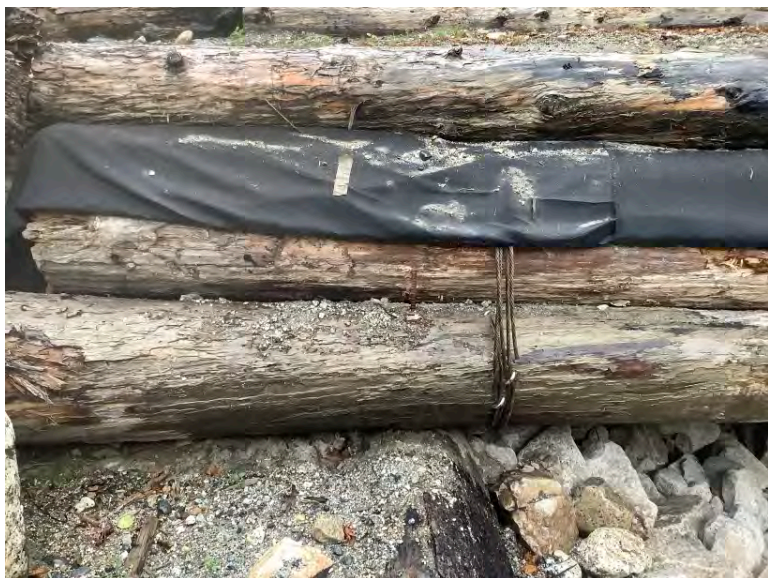
Outside stringer tied to sill
