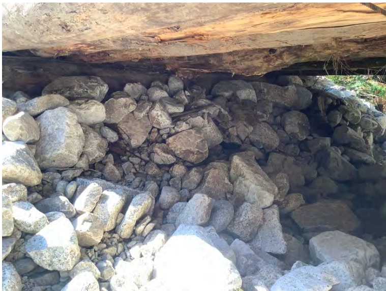
Left Bank Abutment when facing downstream
