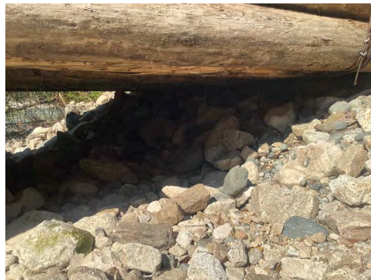
Right Bank Abutment when facing downstream
